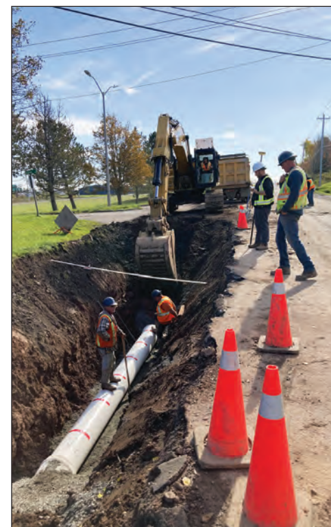
A new 4.5-kilometre pressure main is being installed as part of the Sydney Harbour West Wastewater Collection and Treatment Project.
