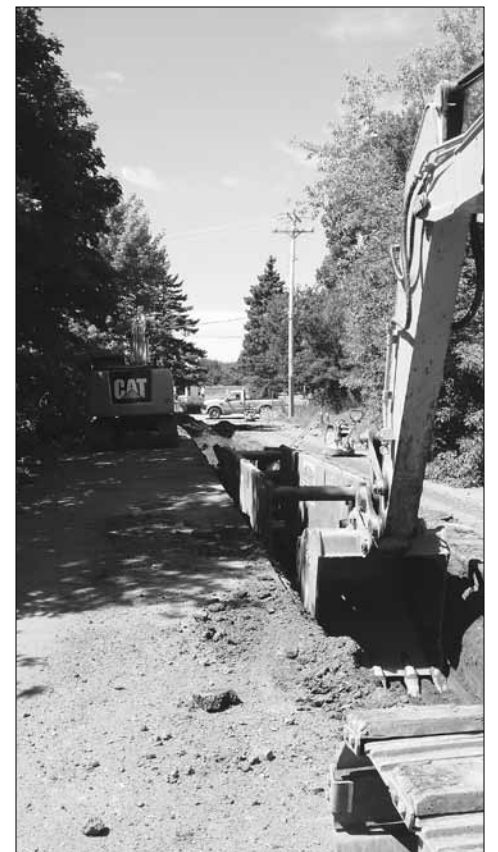
The new water system includes the installation of 30 kilometres of piping.
