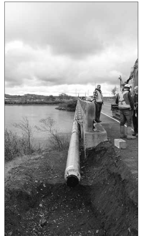
The new piping being installed is a combination of PVC and DR 18.
