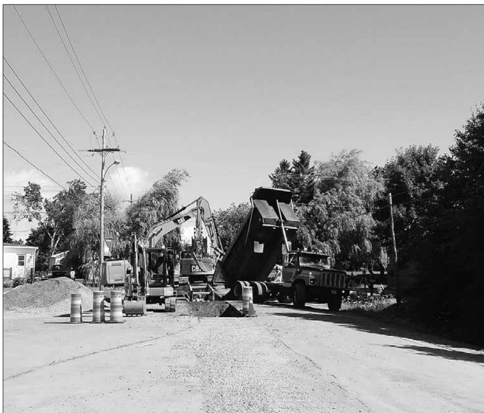
About 90 per cent of the piping has already been installed, with the remainder expected to be completed by summer’s end.
