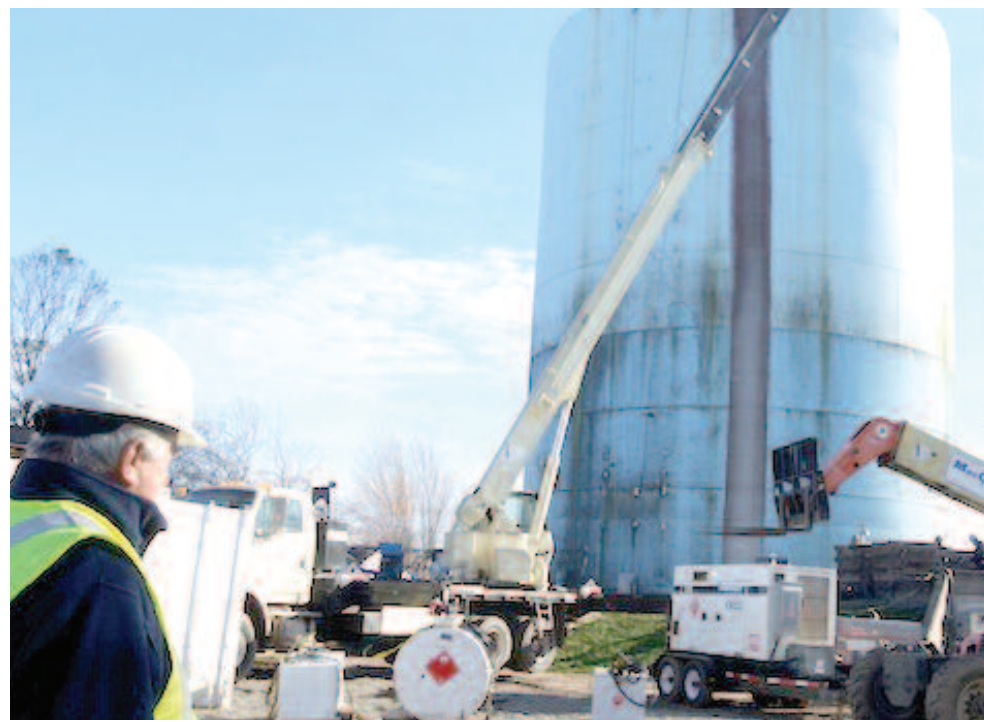
Pictou town engineer Jim Chisholm monitors the work taking place on the Nova Scotia town's water tower. The work is expected to last at least five weeks and alternative plans are in place to supply residents with water during this time. (Photo: Sueann Musick/The News)
