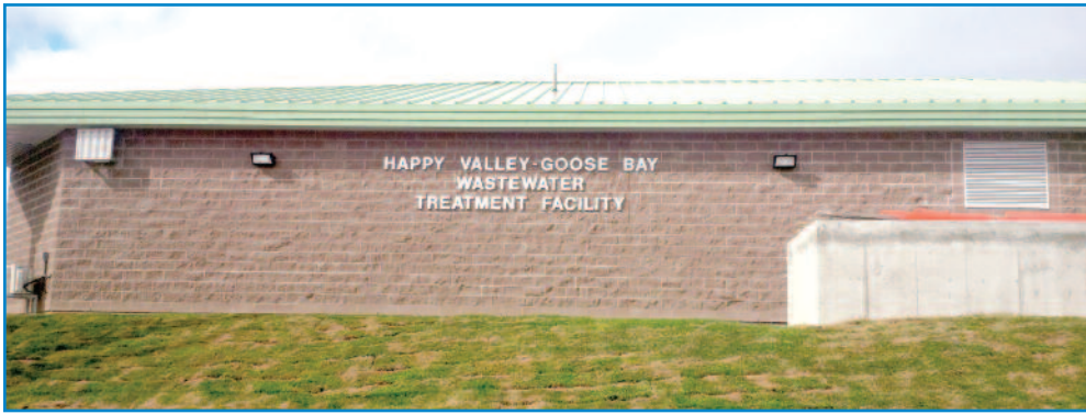
The Happy Valley-Goose Bay Wastewater Treatment Facility opened Oct. 24. (Photo: Wayne Wall)
