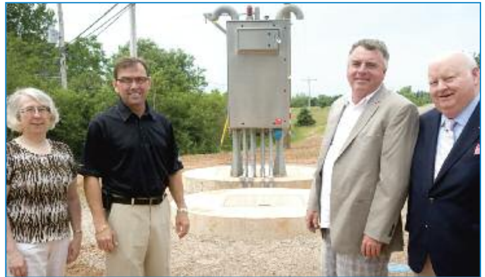
In July, a new water and wastewater servicing system was installed to connect Miltonvale Park to the City of Charlottetown's utilities. In the photograph Miltonvale Park Council Chair Betty Pryor; Prince Edward Island Transportation and Infrastructure Renewal Minister Robert Vessey; Miltonvale Park Councilor Hal Parker, and Senator Mike Duffy view Miltonvale Park's new system. (Photo: Brian Simpson, PEI Provincial Photographer)
