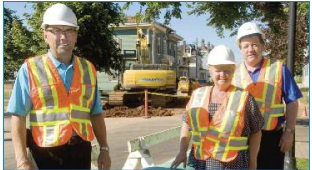
Prince Edward Island Transportation and Infrastructure Renewal Minister Robert Vessey, Minister of National Revenue Gail Shea and Charlottetown Mayor Clifford Lee tour construction of the Spring Park sewer separation project. (PEI government photo: Brian Simpson)
