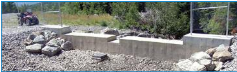
The water supply servicing the town of McIvers, Newfoundland & Labrador was bone dry until workers removed obstructions preventing water from feeding into the reservoir July 16. (Photo: Submitted to the Western Star )
