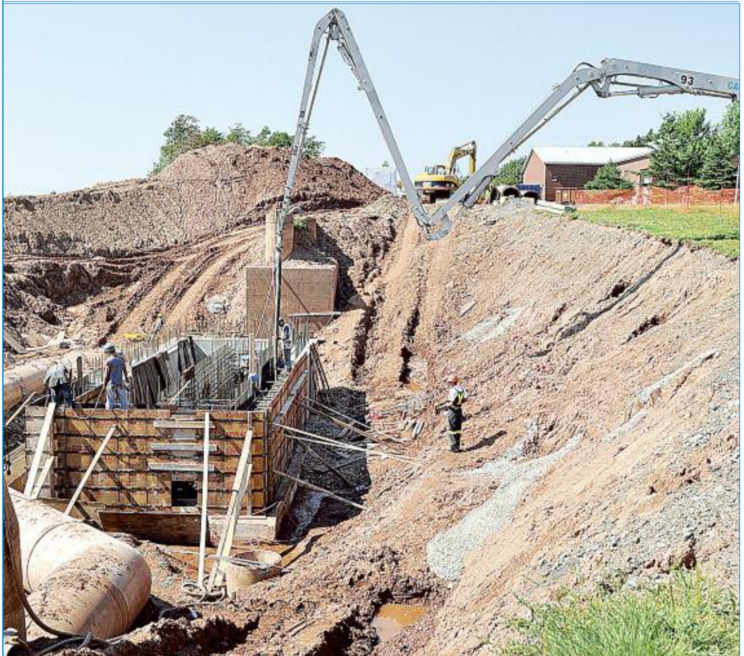
Construction workers are in the process of completing work to the screen tank that will receive raw sewage at the municipal wastewater treatment facility in Lower Truro, Nova Scotia. New systems are starting to come online and the entire process is expected to be up and running by December. (See the story on page 8.) (Photo: Harry Sullivan/Truro Daily News)
