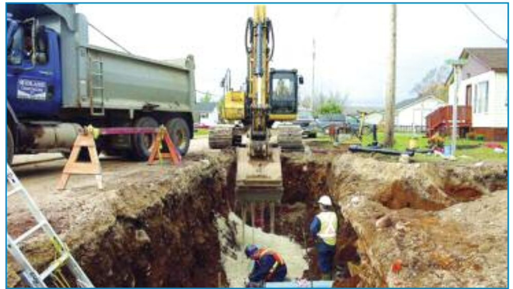
Workers laboured to finish the water and sewage upgrades in the area of Colbourne and Birch streets in Deer Lake, Newfoundland & Labrador. Brendan Bonia, left, and Shawn Durdle worked in the hole while John Maxwell operated the excavator. (Photo: Paul Hutchings/Western Star)
