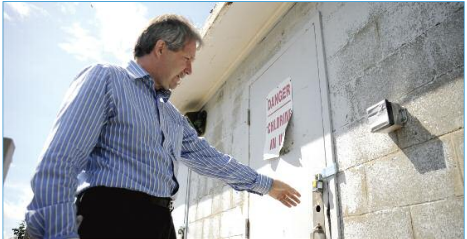
Harbour Grace Mayor Don Coombs inspects some of the damage done to the Newfoundland & Labrador town's water treatment facility on Bannerman Lake Road in late May. It is estimated that the vandals did some $20,000 worth of damage to the facility. (Photo: Nicholas Mercer/The Compass)
