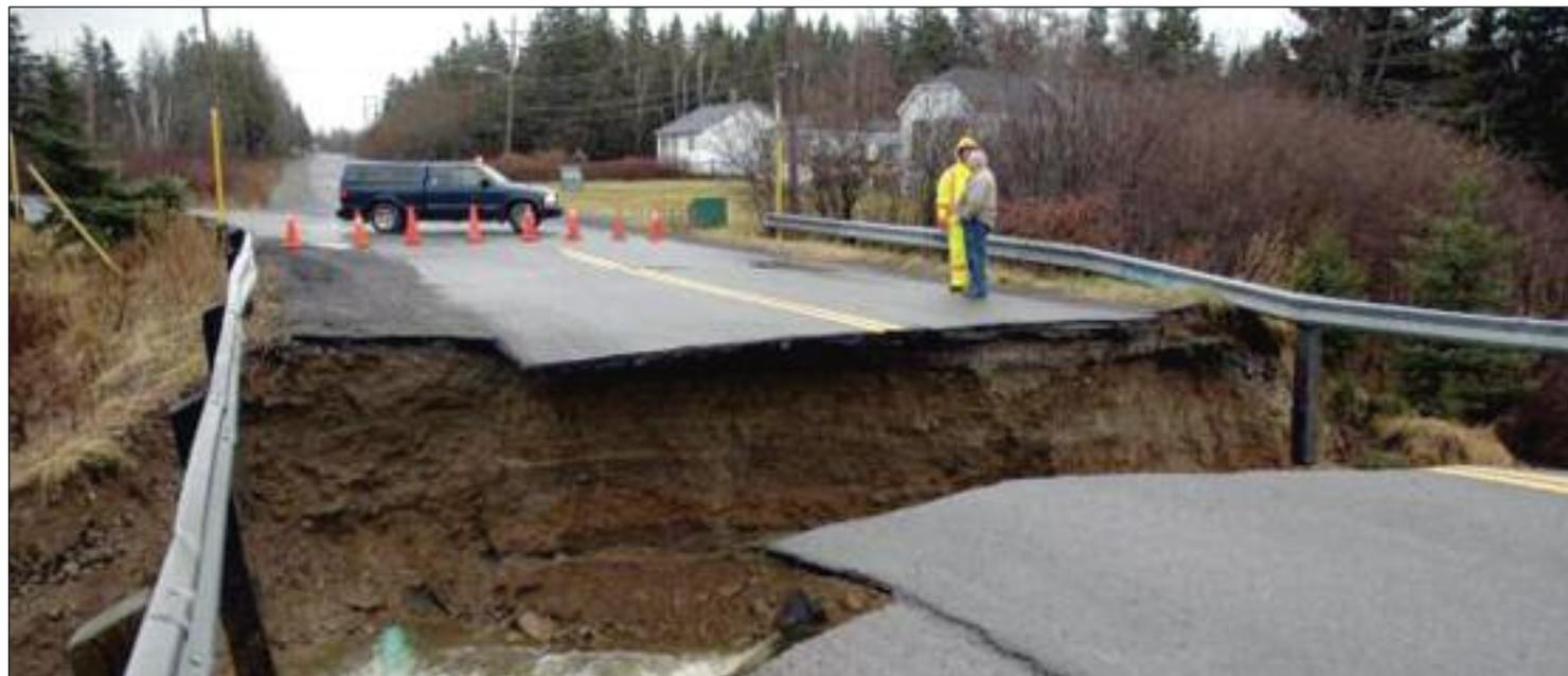
Work began Dec 22 to replace the sewer line on Villa Drive on the Northside of Cape Breton to shore up the water main, replace the culvert and repair a 20-foot gap in the road caused by the week’s heavy rains. (Photo: Julie Collins/ Cape Breton Post)
