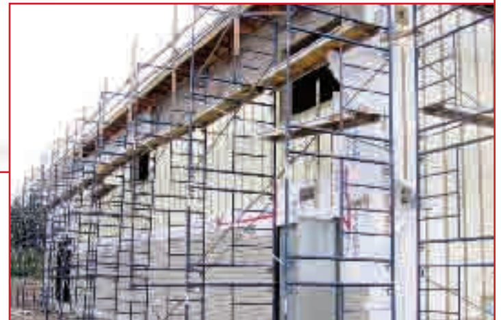
The six-year project included the design and construction of a new water treatment plant, a treatment process waste disposal system and upgrades to the transmission and storage facilities.
