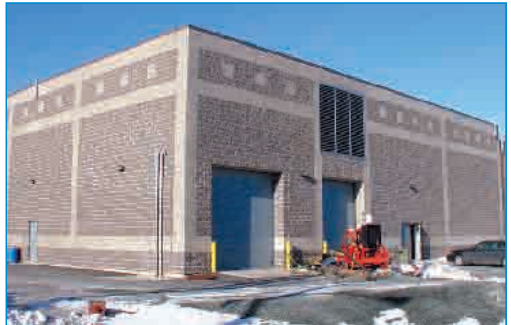
The municipality is hoping to have the Halifax WWTF fully restored by spring 2010.
