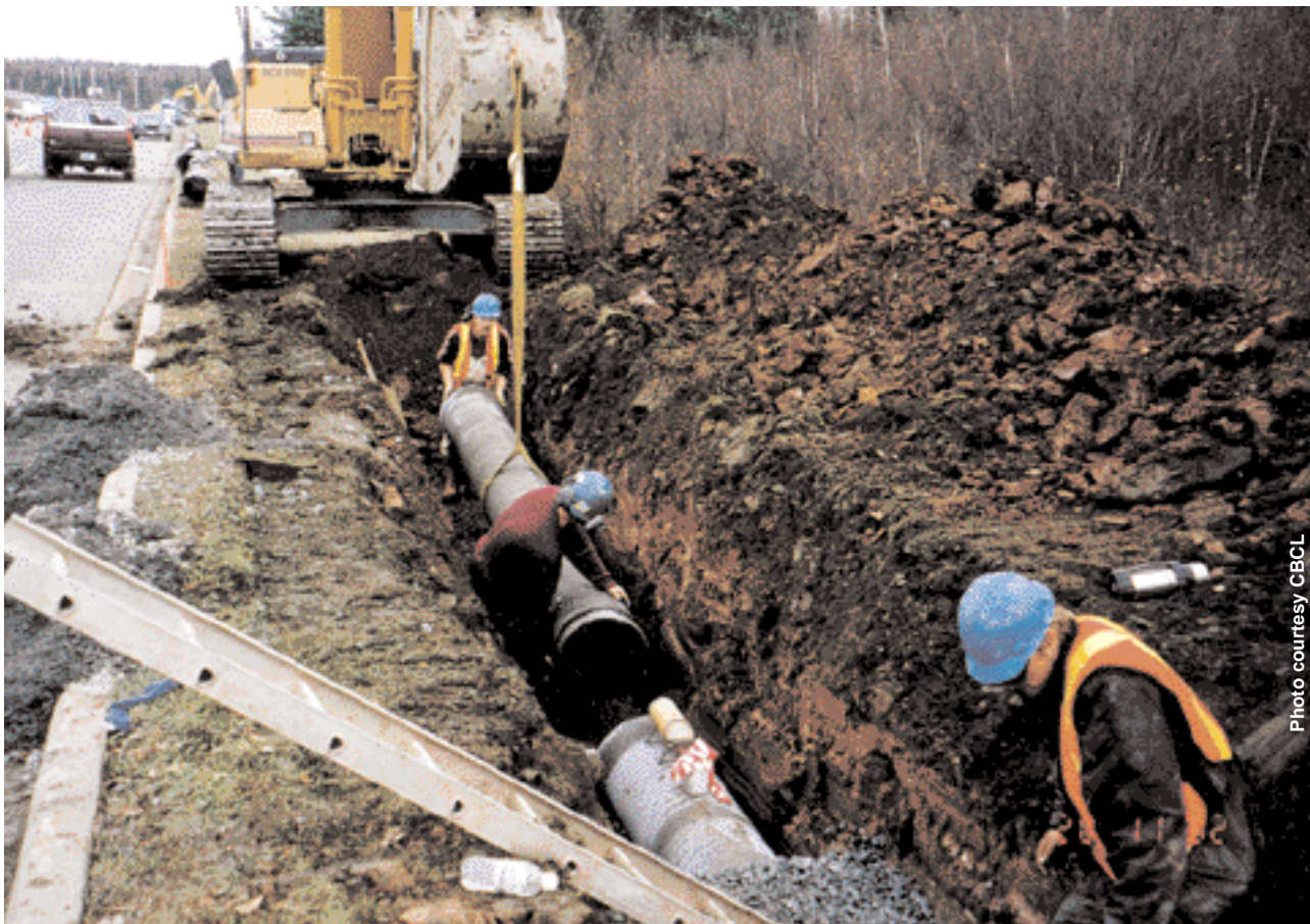
A 16-inch high-flow water pipe is installed along Bell Boulevard in the spring. Upgrades under Phase 2 were the extension of the main along Bell Boulevard to the existing HIAA water reservoir, the completion of the loop from the airport's reservoir to the north end of the terminal building, and replacement of existing old water lines around the main terminal building. Upgrades also included replacement of the old water line along Barnes drive and replacing existing services along those lines — all new hydrants and service lines.
