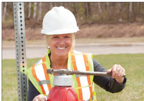
Valérie Michaud is a water and sewer operator for the City of Dieppe.
