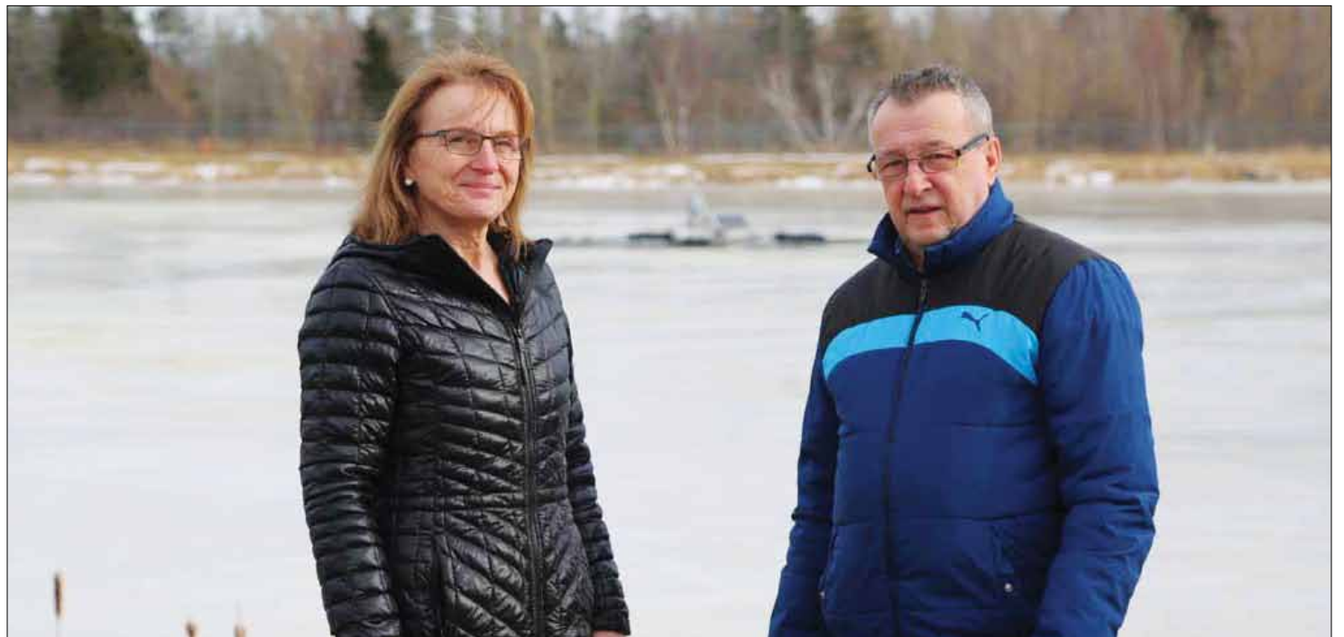
Georgetown CAO Dorothy MacDonald and Mayor Lewis Lavandier stand in front of the new lagoon that now services the town of 550 people. The lagoon was built using joint funding from the Clean Water and Wastewater Fund.
