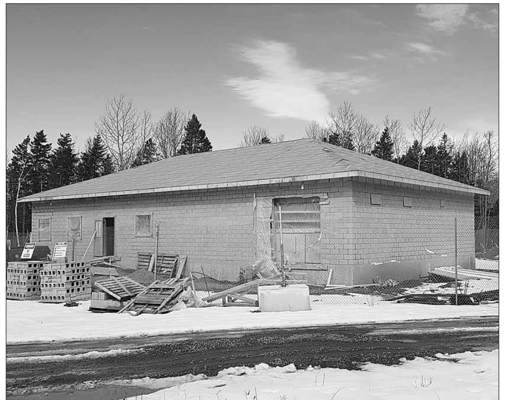
The water treatment facility currently under construction in Pictou.
