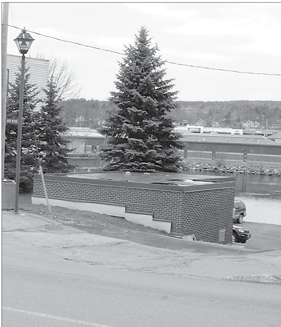
Pump station 4 in Bridgewater. A failure in the main discharge pipe this past February proved to be a challenge to repair.
