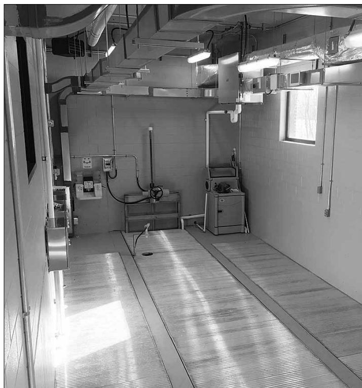
Looking back the other way at the discharge end of the UV building, you can see the sampling and control equipment in the background.
