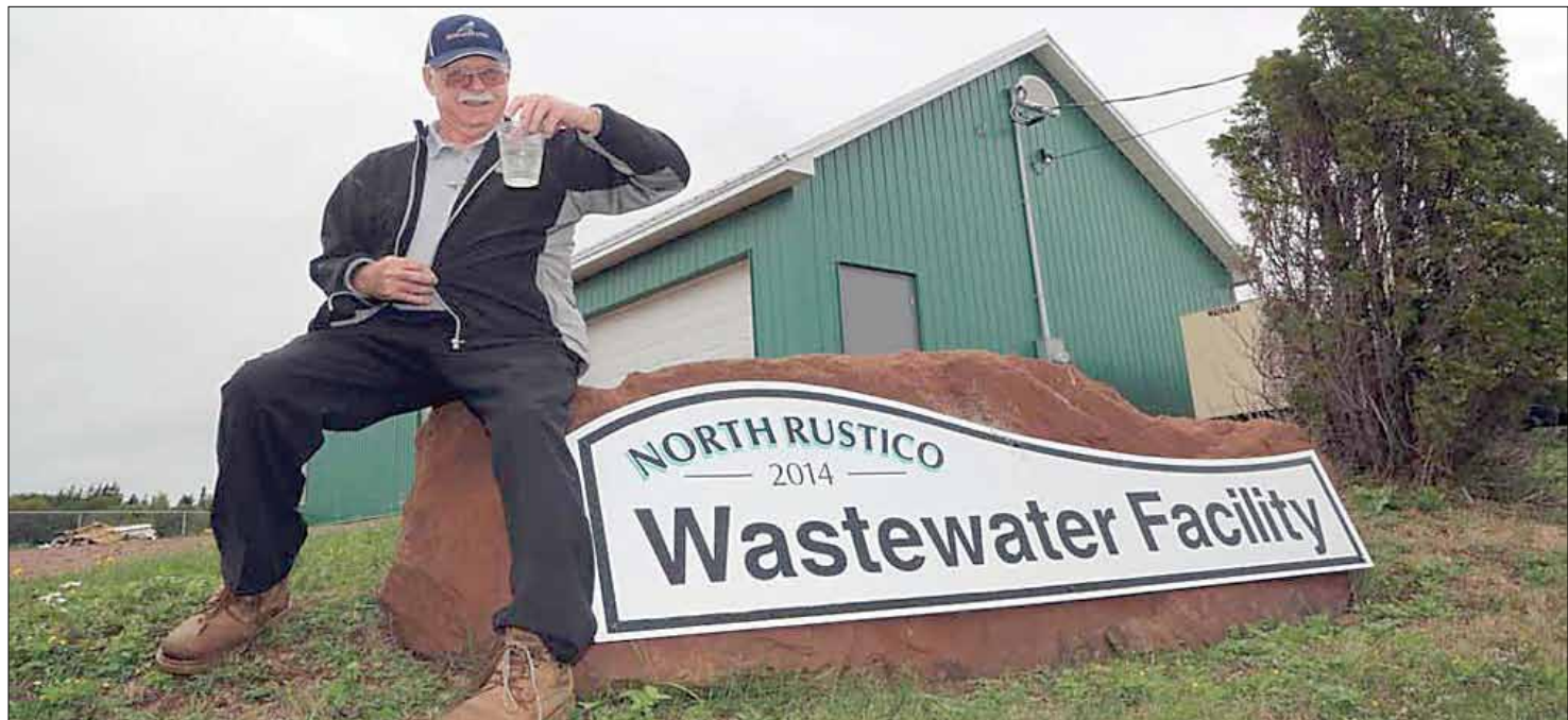
Les Standen, chair of the North Rustico Water and Sewer Committee, holds up a glass of clear effluent from the town's wastewater facility. Submitted photo
