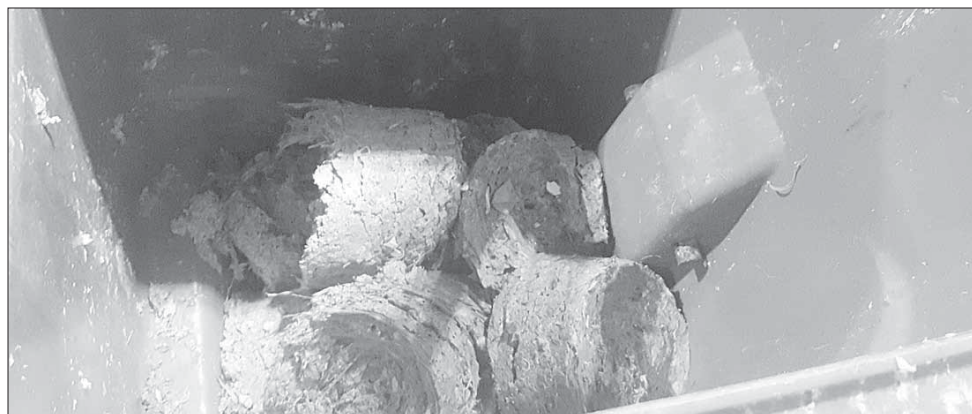
Non-organic material (plastics, rags, etc.) captured by the screens is then compressed to remove the liquid and then directed into green bins. In the summer the volume captured daily amounts to approximately half a green bin.
