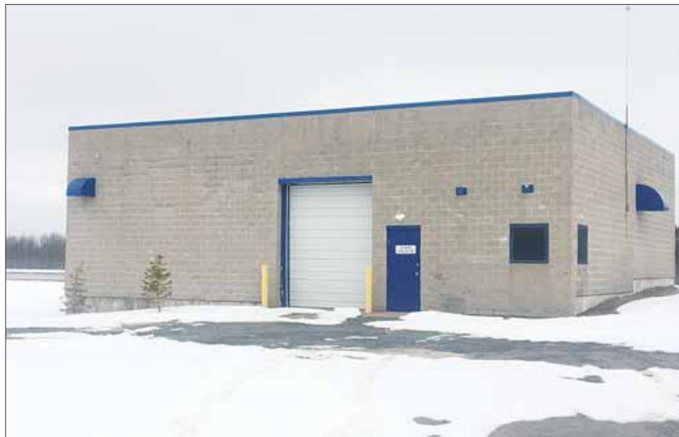
Springhill’s current wastewater system, housed in the building shown above, is “relatively new” at just 30-years-old, says Justin Waugh-Cress, director of engineering and operations for the Municipality of Cumberland. It’s the 60 to 100-years-old pipes that need to be replaced.
