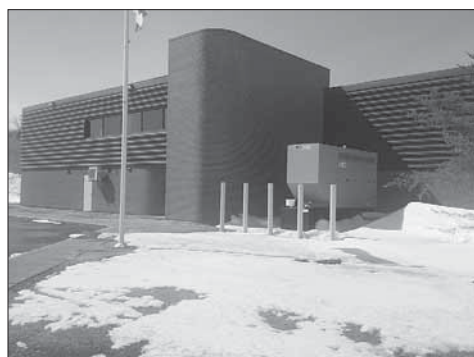
Another portion of the project involved the installation of an exterior genset 300 kilowatt generator, which will provide power to the entire wastewater treatment facility in the event of power failure.
