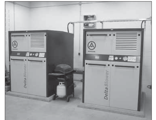
The new system meets the regulatory standards set by the New Brunswick Department of Environment and Local Government, requires less maintenance and is more than 25 per cent more energy efficient than the previous system.
