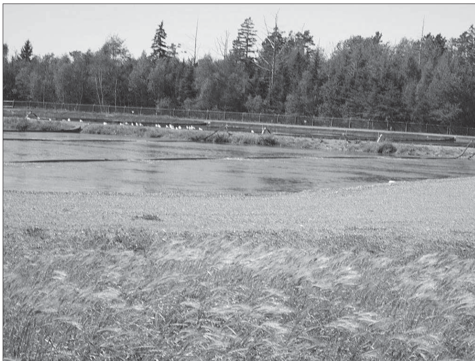
To save on costs and reduce land usage, the town opted to re-line the previously existing lagoons, which are now dredged periodically.
