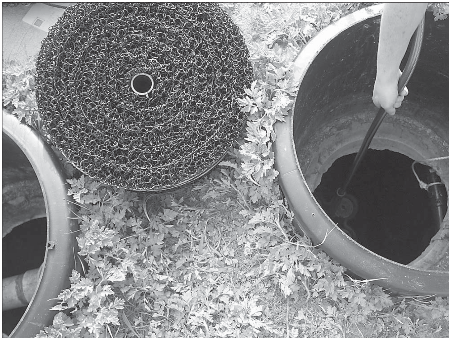
The residential ClearPod solution being installed on an existing treatment system.
