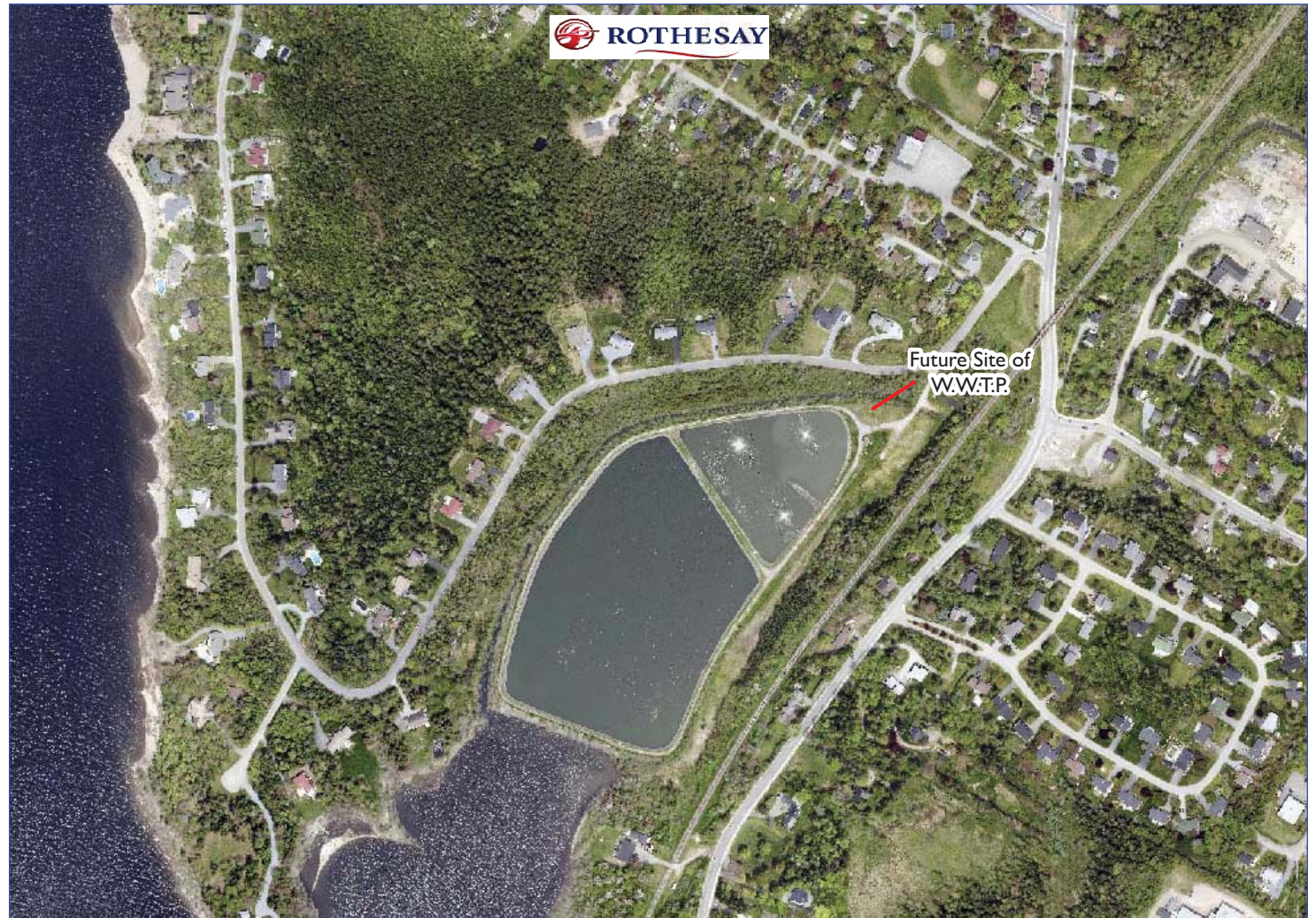
Rothesay's Sagamore Point wastewater lagoon will also be the site of the town's new treatment plant. Two other lagoons will be phased out as the new system is brought online. (Supplied Photo)
