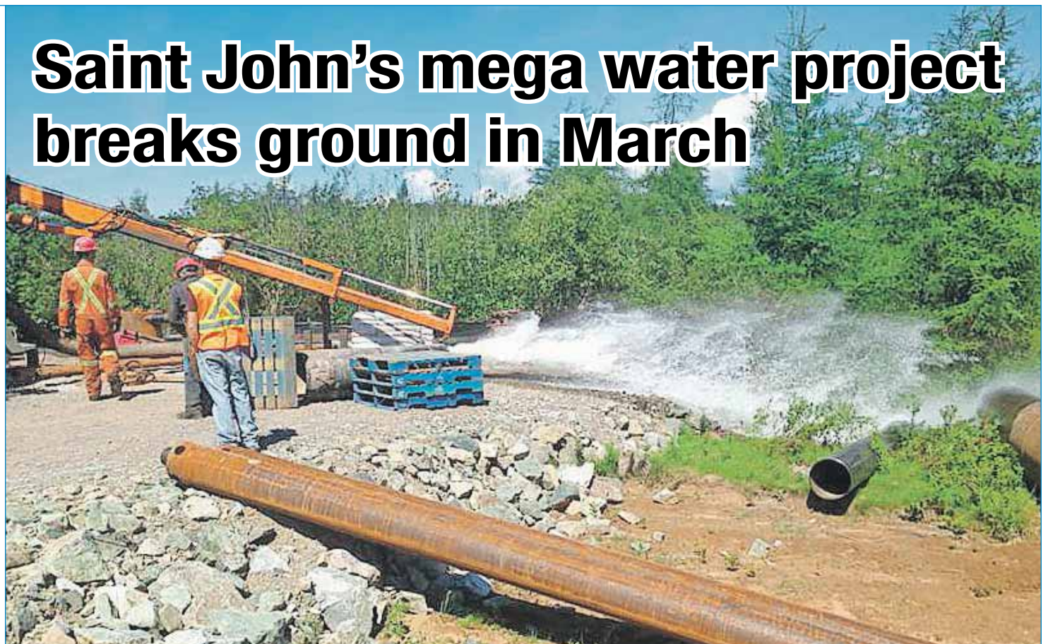
Workers clean and develop production wells that will supply the Saint John's West side with drinking water once the city's new water treatment plant is completed. - Submitted photo
