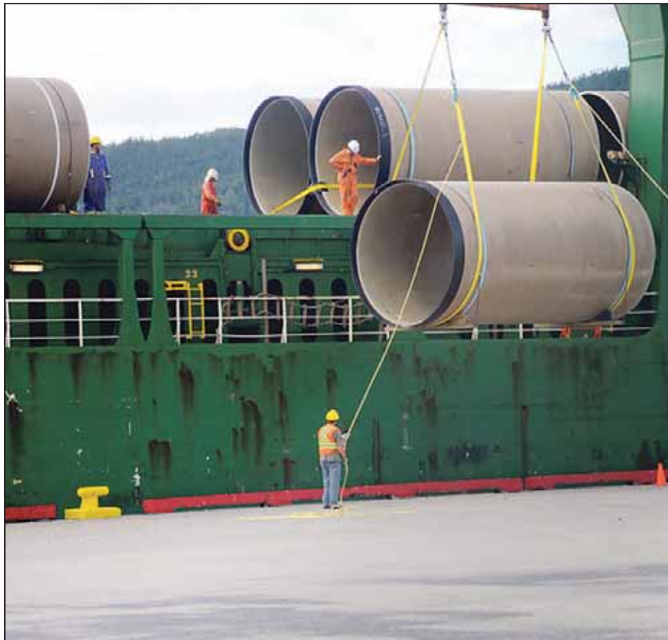
Pipes destined for Deer Lake Power to replace the penstocks were off-loaded at the Corner Brook Port on Aug. 15. (Photo: Cory Hurley/ Western Star)
