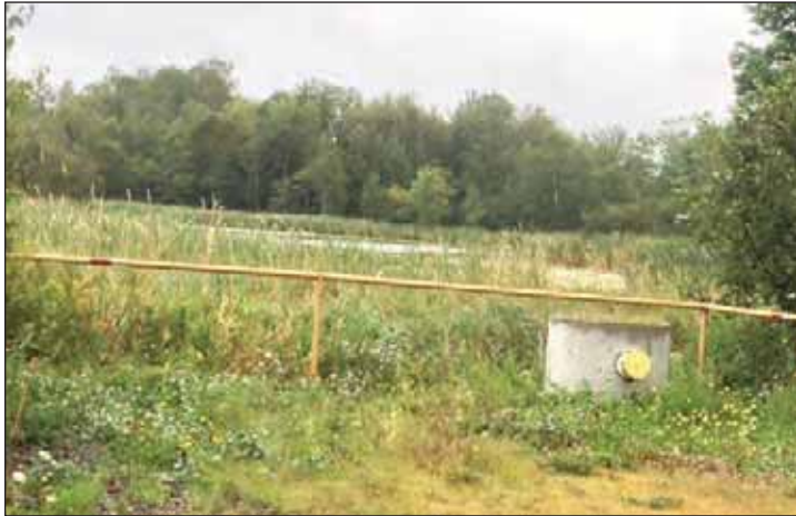
Berwick's fire department is getting three new dry hydrants at ponds on the north mountain in order to improve service to Berwick's outlying communities. (Photo: © Nancy Kelly/Register/Advertiser)
