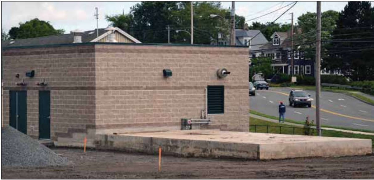
The greater Sydney wastewater collector project was recently completed. The $15.3-million project directs sewage outfalls for treatment. (Photo: Greg McNeil/Cape Breton Post)
