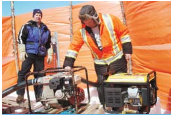
St. Anthony Bight residents Walter White, left, and Wayne Taylor take a shift pumping water from Big Brook Pond to the Newfoundland & Labrador community's water supply, some 1,400 feet away. (Photo: © Adam Randell/Northern Pen)
