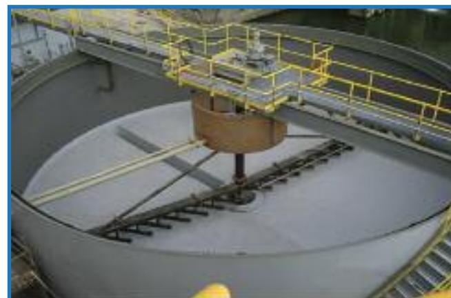
Clarifiers used in wastewater treatment are often designed with metal sidewalls resting on a concrete base. In an attempt to prevent leaks when the concrete base cracks, a unique elastomeric liner is used that “bridges” structural cracks up to one-eighth of an inch and resists harsh chemicals used in wastewater treatment.
