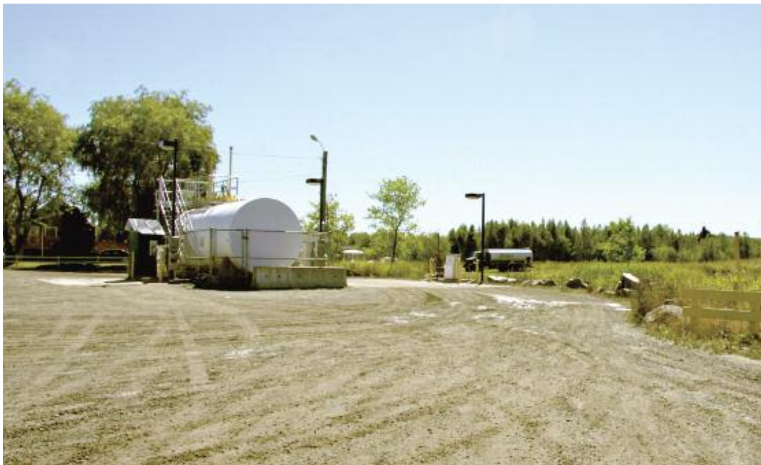
According to Municipality of West Hants, a sinkhole has been developing for about a year near the Oulton's Card Lock Fuel Station.
