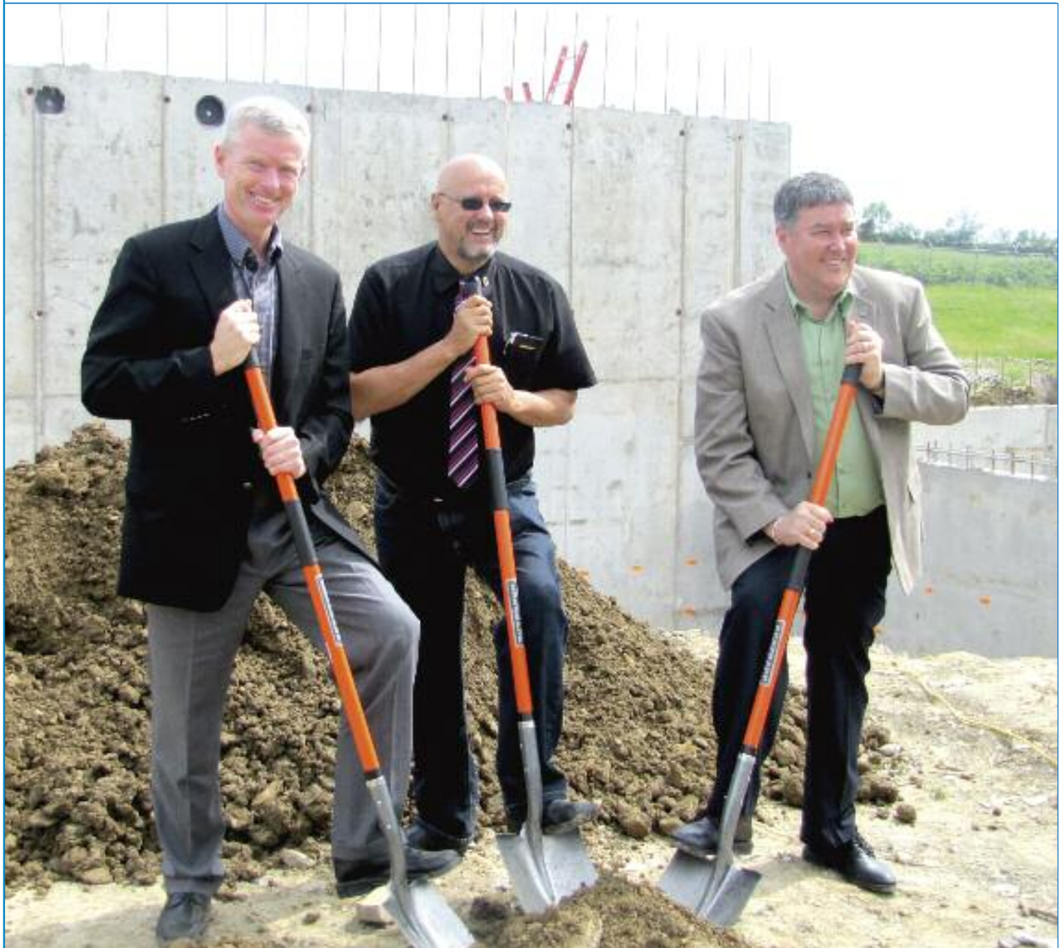
Construction officially began July 2 on the new wastewater treatment facility in Saint-André, New Brunswick. The federal, provincial and municipal governments are each investing close to $1.9 million in the project. In the photo are: Tobique-Mactaquac MP Mike Allen, Saint-André Mayor Alain Desjardins and the NB Post-Secondary Education, Training and Labour Minister Danny Soucy. (Photo: Communications New Brunswick)
