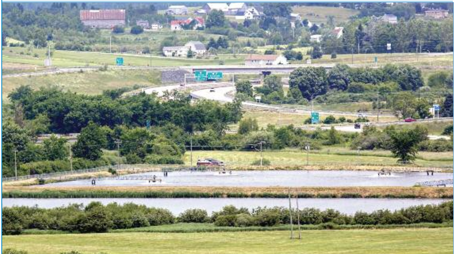
Close to $9,000 has been allocated by Sussex Town Council for yearlong quality tests at its wastewater treatment plant. Crandall Engineering advised council that one sample of the treated water that flows from the plant into the Kennebecasis River had failed. The company recommended that more testing be conducted to determine if contamination was involved or a more serious problem warranted attention. The wastewater treatment plant (foreground) is located just outside the New Brunswick town's western boundaries, beside the Kennebecasis. (Jamie Roach photo)
