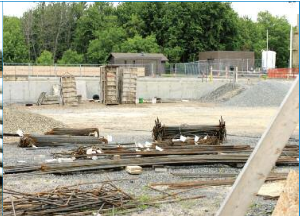
In June Philson Ltd. was working on Phase 1B Upgrades to the Fredericton Area Pollution Control Commission's Wastewater Treatment Facility to accommodate a secondary treatment plant expansion. The project includes construction of a new aeration tank. The Hanwell, New Brunswick sewer contractors (with CBCL as consultants) will also install piping, valves, a blower, pumping equipment and aeration diffusers. (Photos: Heather Jones)
