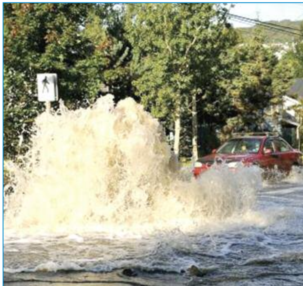
On Sept. 22 vehicles had to navigate around the water gushing up from a water main pipe beneath Mount Bernard Avenue in Corner Brook, Newfoundland that broke shortly after 9 a.m. City Water and Sewer Superintendent Keith Costello said "the west side water feeder main split about 10 feet along its length from a valve to the T-joint where it originated." Water from the Curling watershed was available to local residents while the repair was completed. (Photo: Gary Kean/The Western Star)
