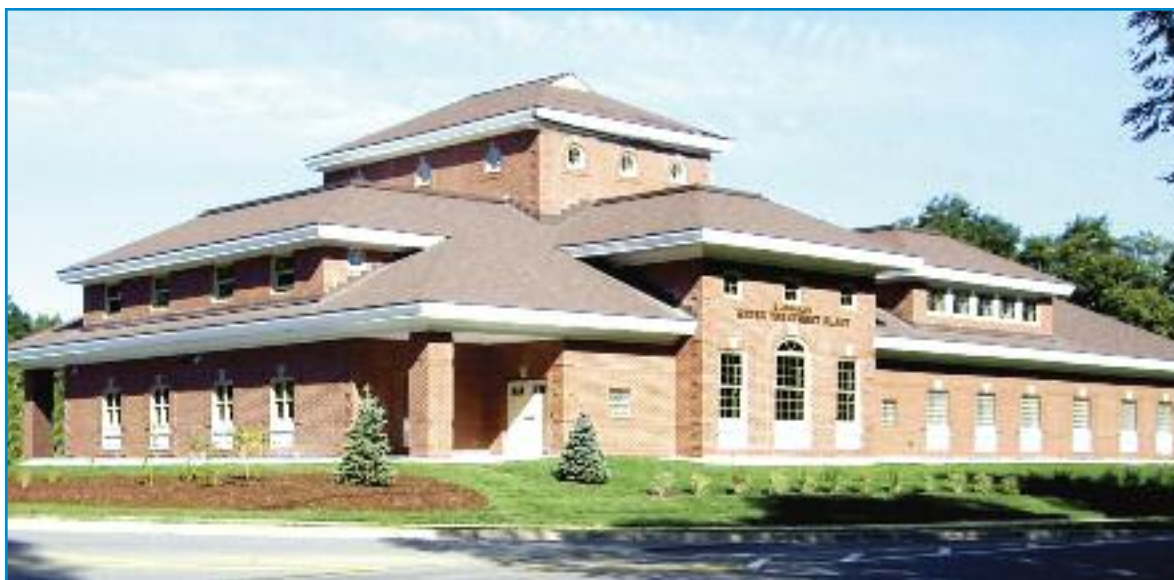
The E. John Bliss Water Treatment Plant.
