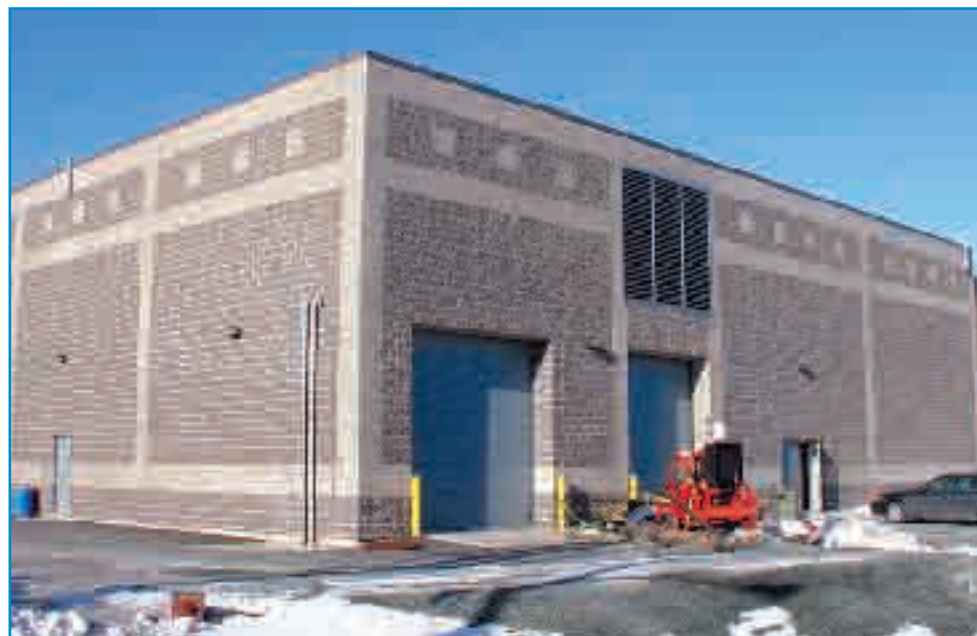
The municipality is hoping to have the Halifax WWTF fully restored by spring 2010.
