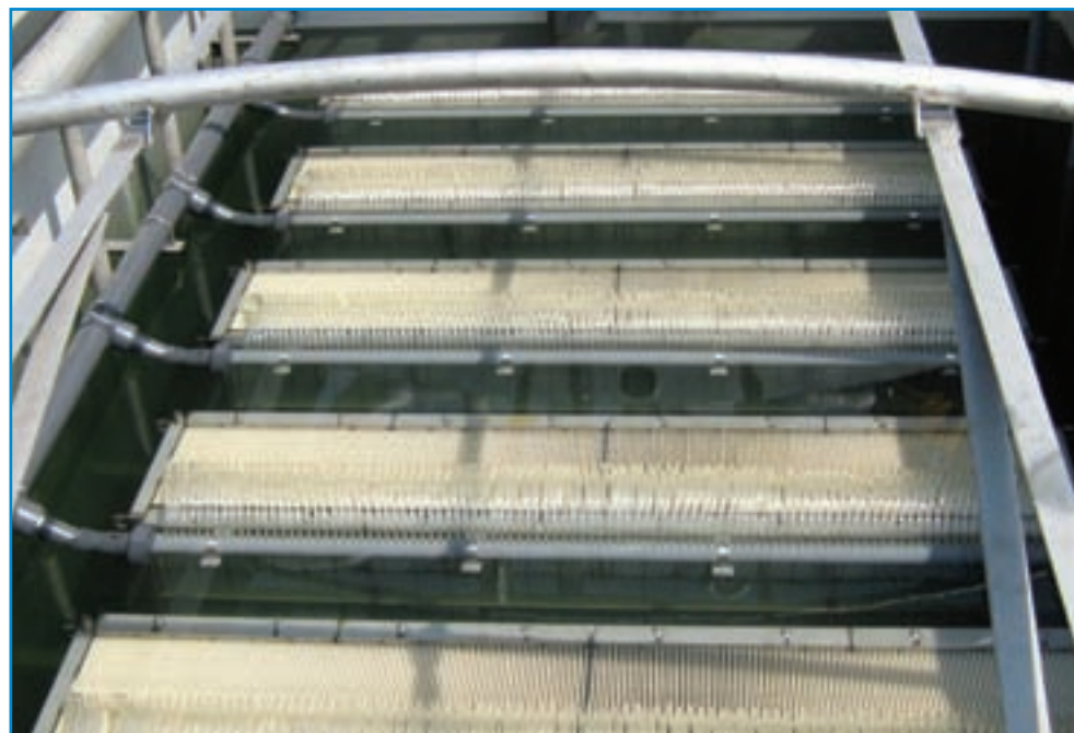
Photo courtesy of ADI Systems Inc. Some of the benefits of ADI's MBR technology include the ability to meet stringent effluent limits, ease of operation, and minimal membrane cleaning.
