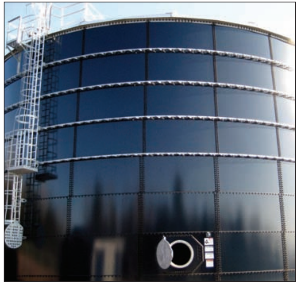
The new 3,500 cubic metre tank features glass-fused-to-steel construction.
