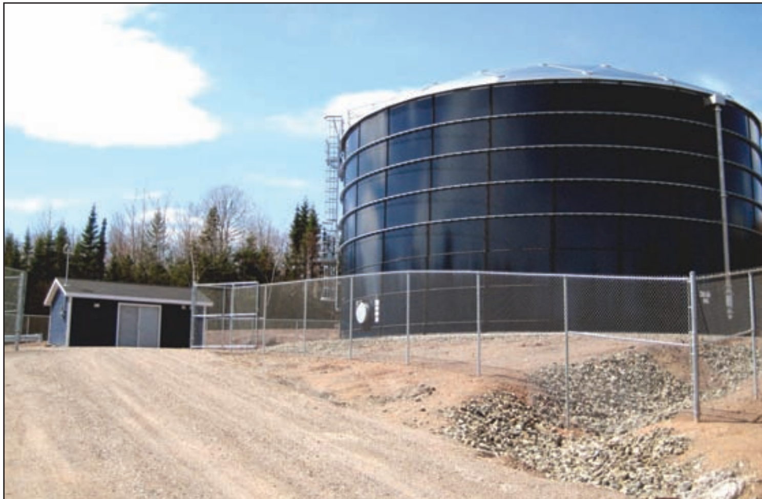
The Wagmatcook project included a new reservoir and new pipes and water lines.
