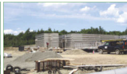
Construction photos courtesy of Dillon Consulting Ltd.
